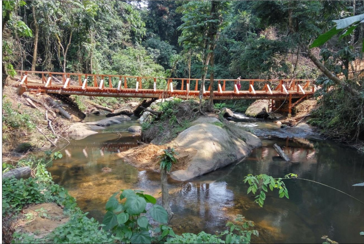
Figure 5.3 Bridge over Biruwe River on Bisie access road
