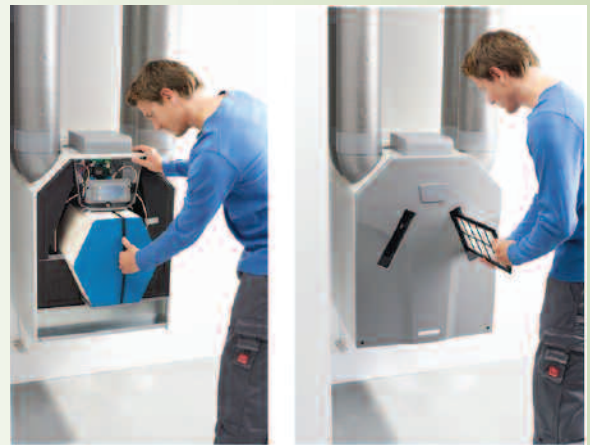
Cleaning the heat exchanger
