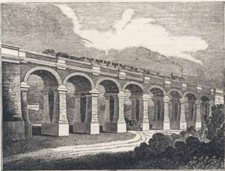
THE WHARNCLIFFE VIADUCT
