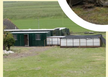
Quarantine unit in place at the Project Site
