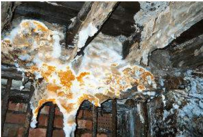
A further feature of the fungus is the formation of 'strands', thick walled structures which develop in the fungal growth. These are resistant to desiccation and carry nutrients from the food source to the growing tips of the fungus when the organism is growing through or over nutritionally inert materials, eg, masonry, soil. They support the spread of the growth. However, without a source of food growth is terminated.
