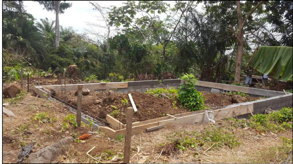
Foundations being laid for the quail farm
