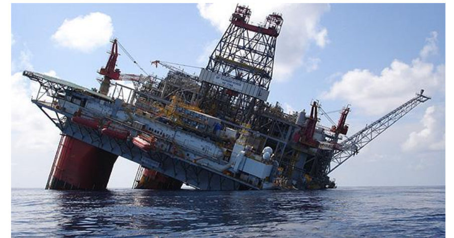
Damage from Hurricane Katrina
