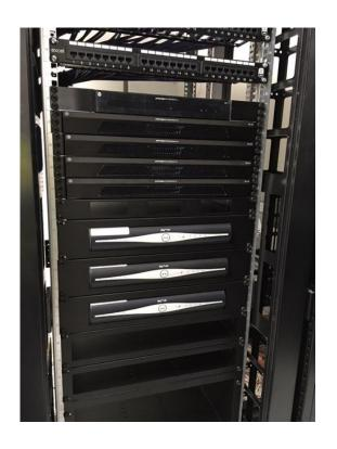
A fully dedicated communications room was designed and installed where all 3 floors of data cabling terminated into.
