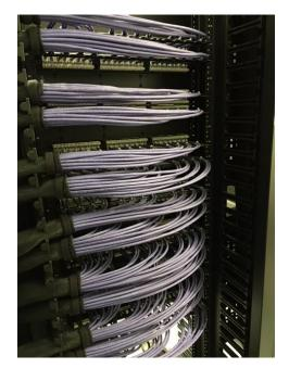
Cat6 data cabling was the basis of the horizontal cabling throughout the offices, run through false floors and along exposed cable tray such was the industrial design setting of the building
