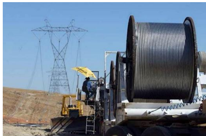
Figure 3.2.5 Stringing Conductor Cables between Towers
