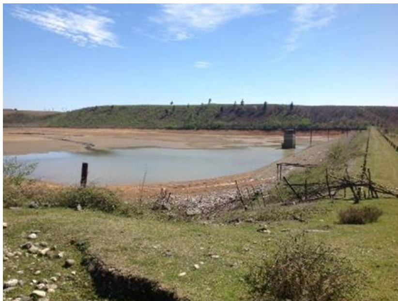
Figure 6.1.3 View of Kukhi Reservoir
