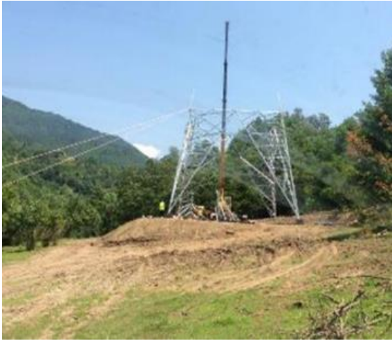
Figure 3.2.3 Tower Assembly Works
