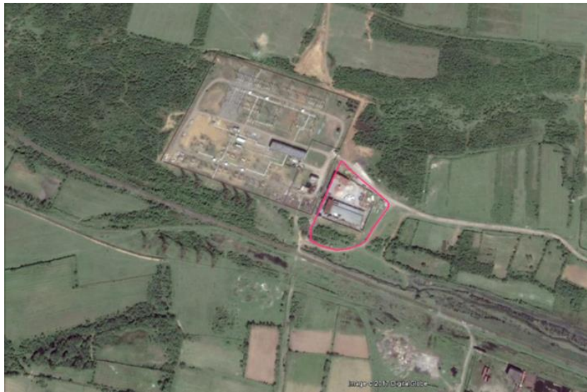
Figure 3.2.7 Indicative Location of Construction Camp adjacent to Existing Tskaltubo Substation
