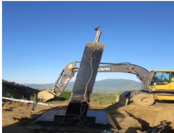
Figure 3.2.4 Installing a Precast Concrete Foundation
