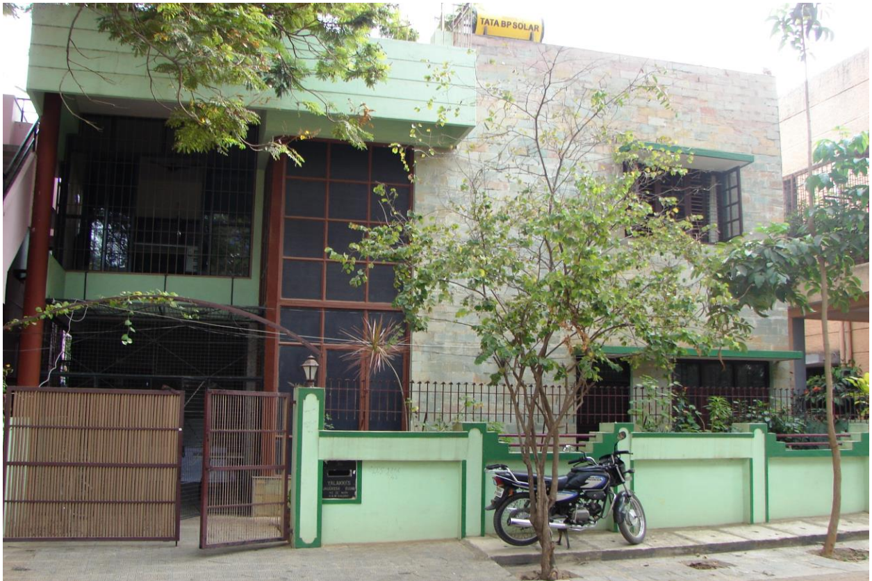
New ASHA Foundation premises
