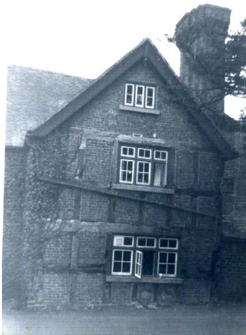
Balderton Hall showing the original end of the Hall
