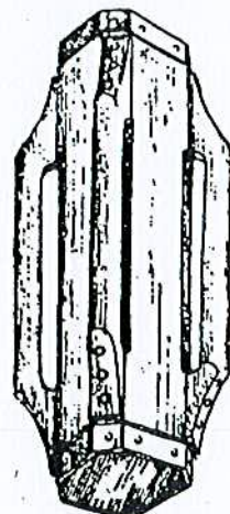
Sometimes a hand-pile-driver was used for a ram (1519).
