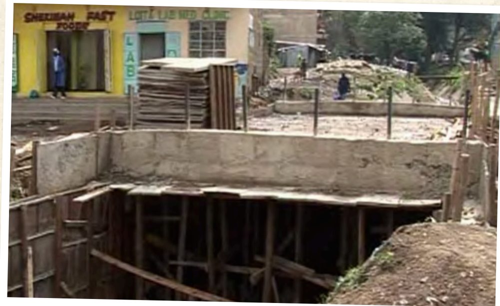
Improved water drainage in Narok town prevent flooding
