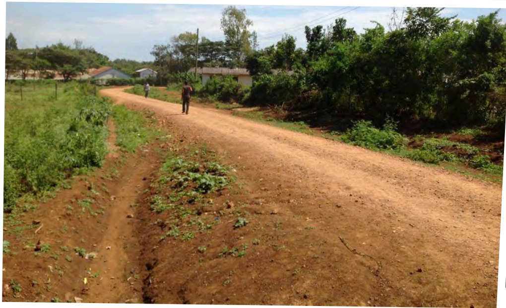
Newly constructed road in Siaya County
