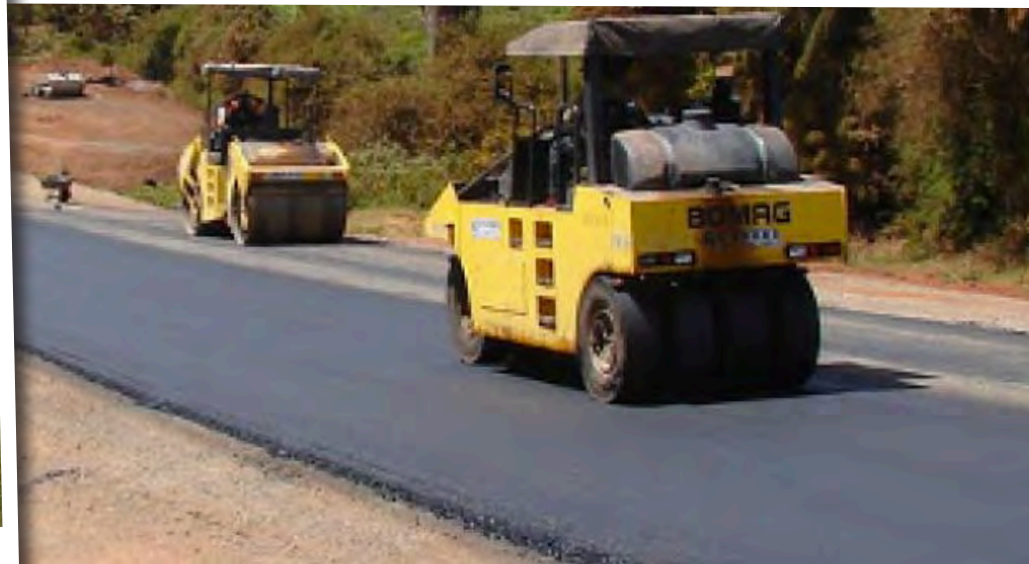
Tarmacking roads in Taita Taveta County
