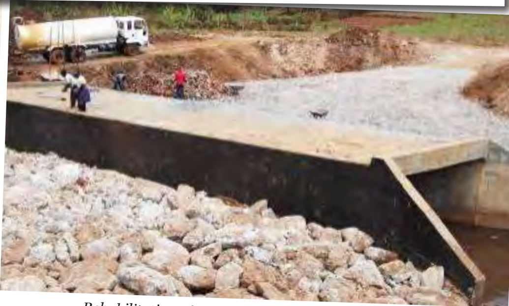
Rehabilitation of Mukuyu-Githambo-Kiruri Road
