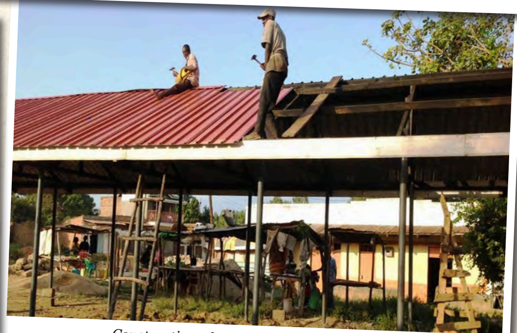
Construction of market shades in Kitui County
