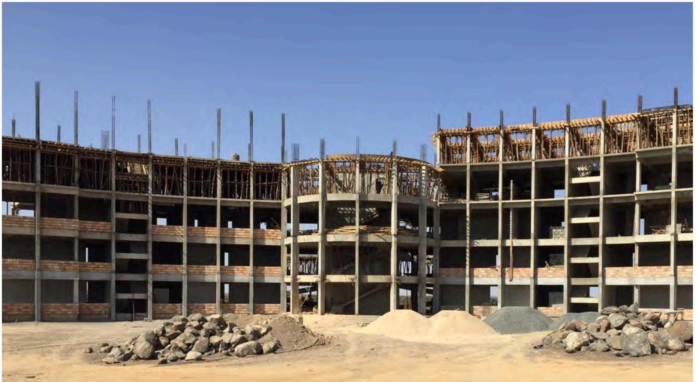
Ongoing construction of Turkana County Headquarters
