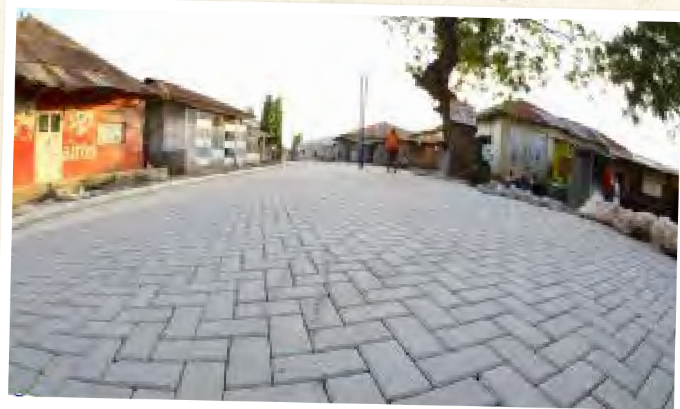
Ongoing Mkomani road paving in Mombasa
