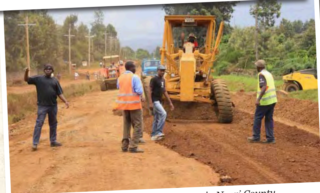
Marua-Nyeri road at Muruguru in Nyeri County
