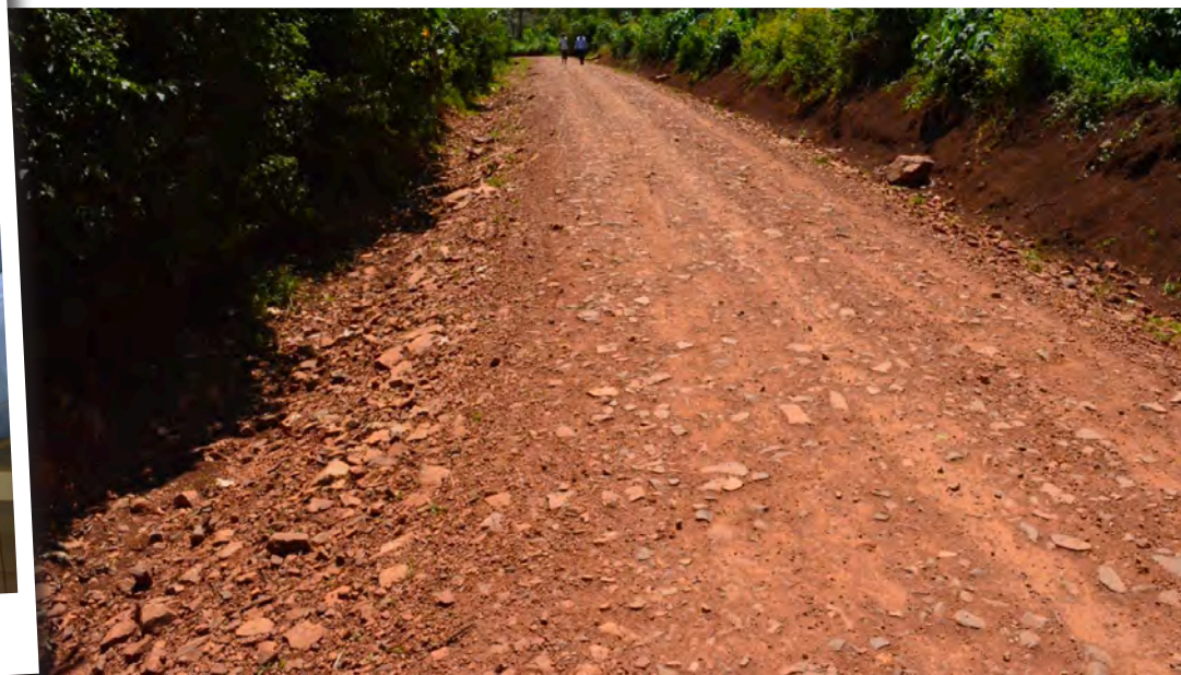
Bombo-Kegogi-Nyamonuri murram road constructed in Nyamira County
