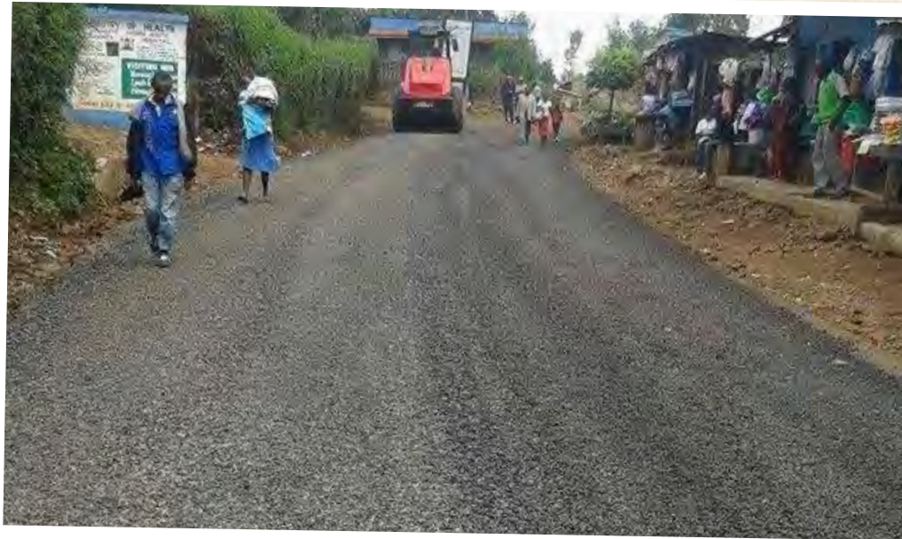
Tarmac road under construction in Maua Town
