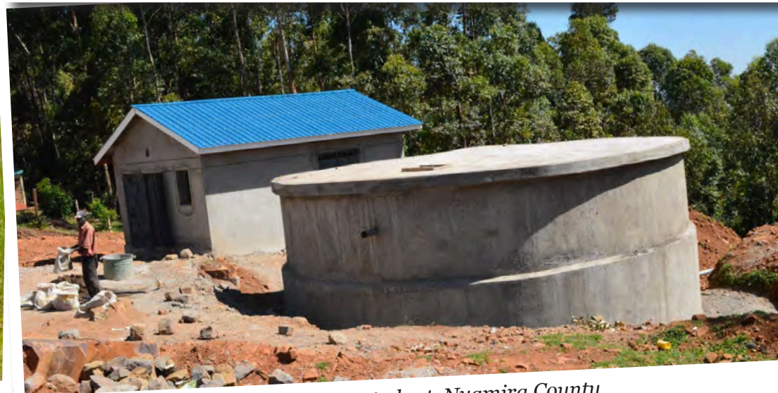
Water treatment plant, Nyamira County
