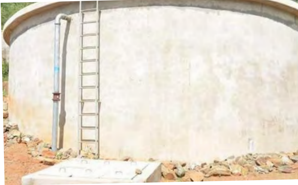
Voi water project, Taita Taveta county
