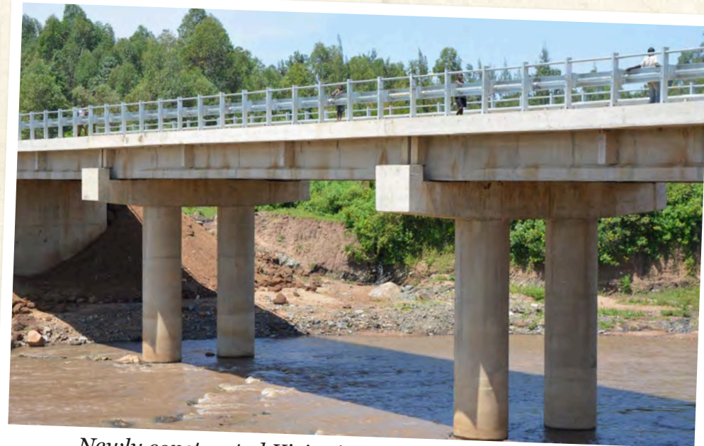
Newly constructed Kiringi Bridge in Migori County
