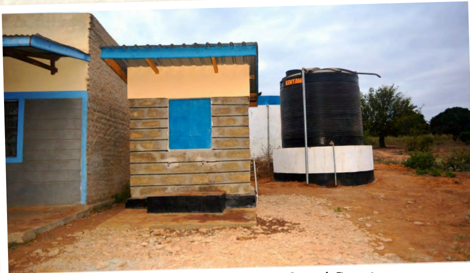
Water kiosk in Nzueni, Makueni County
