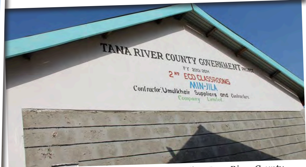
ECDE Classrooms constructed in Minjila, Tana River County
