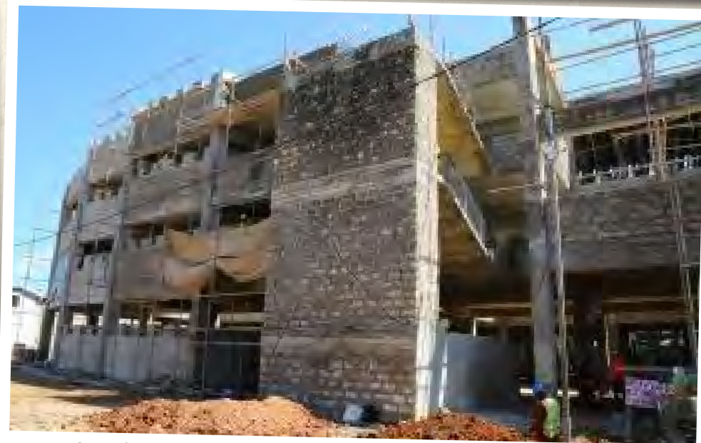
Ongoing construction of Kongowea market block, Mombasa
