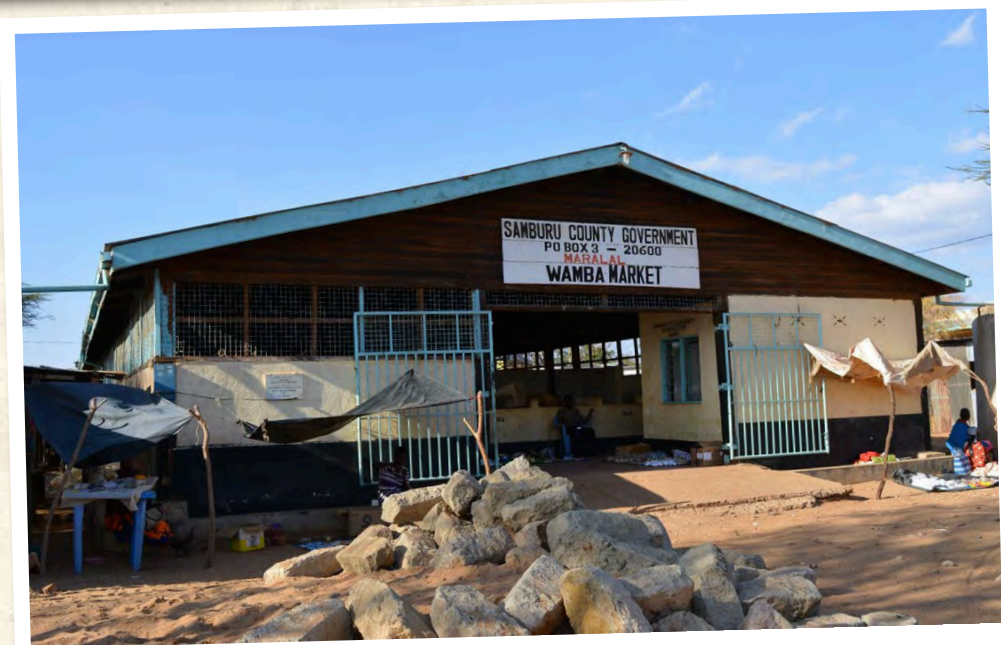
Wamba Market under construction in the county
