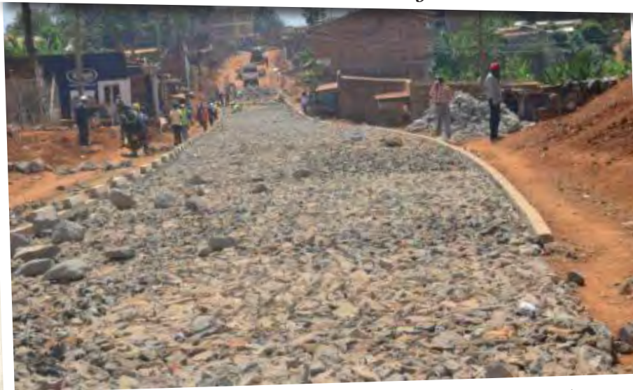
Chuka General Hospital road in process of tarmacking
