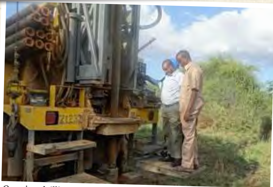
Ongoing drilling of a borehole in Eldas Sub-county, Wajir County
