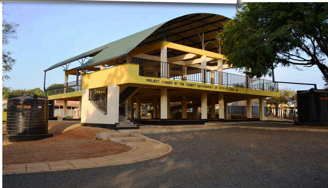
Modern market shed at Matinyani - Kitui County
