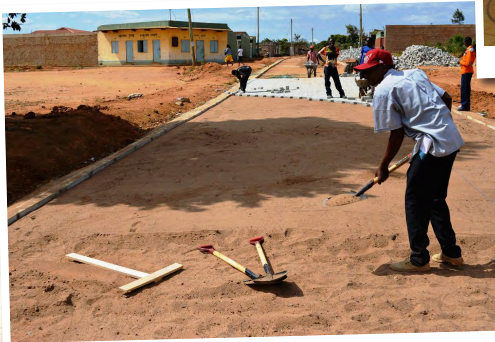
Ongoing road construction in Makueni County
