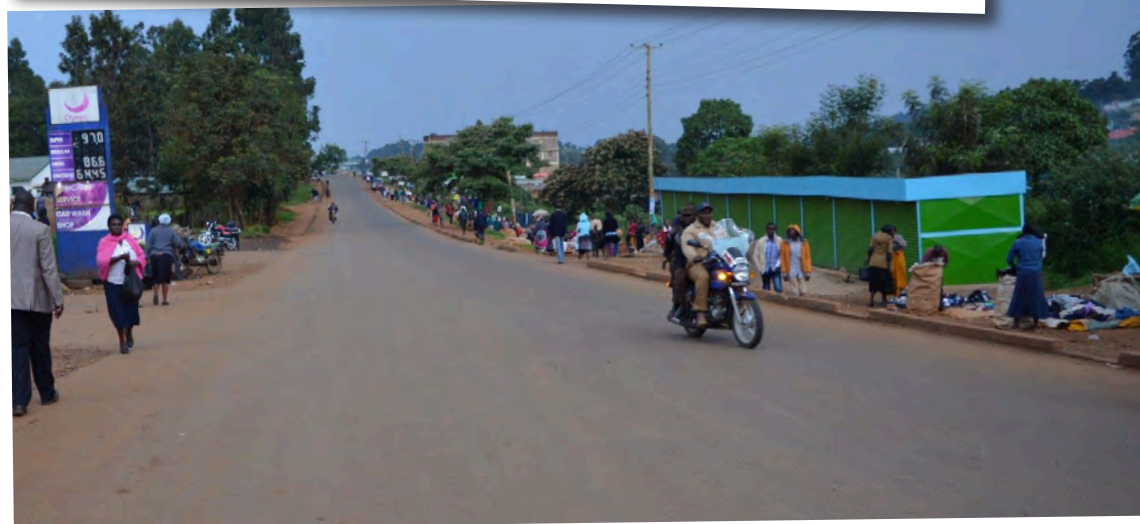
Tarmac Road constructed in Nandi Hills, Nandi County
