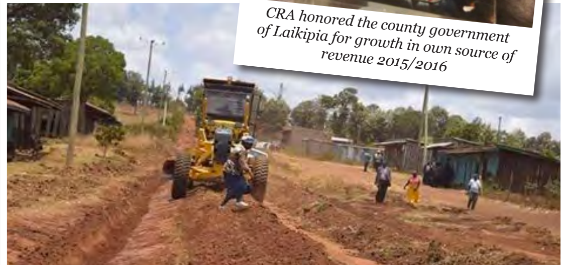
Ongoing construction of roads in Laikipia County
