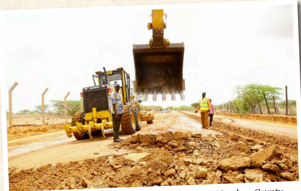
Construction of the main town road, Mandera, Mandera County
