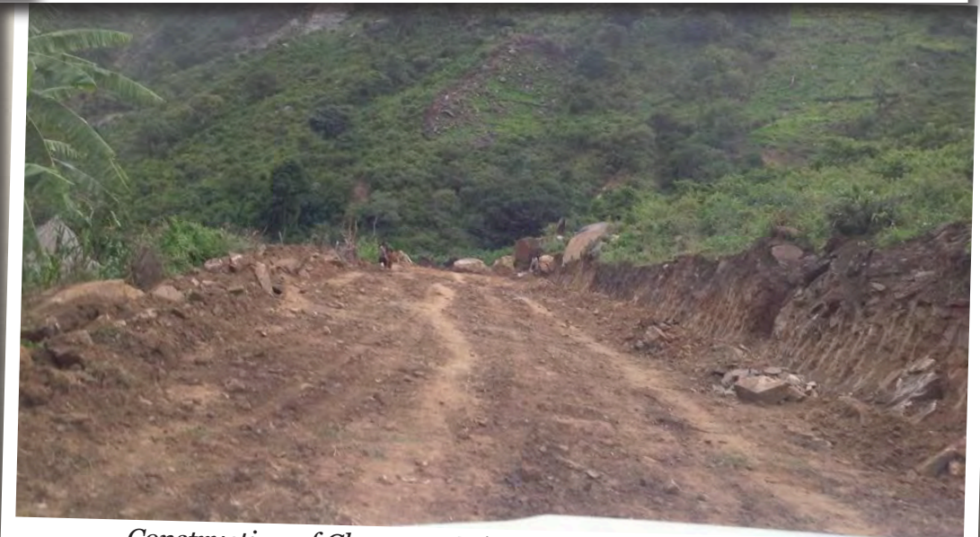
Construction of Chesegon-Ptirap road , West Pokot County
