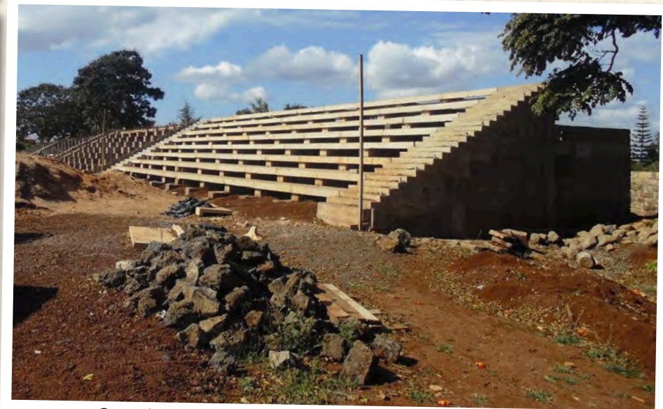
Ongoing construction of Meru Stadium Meru—2015
