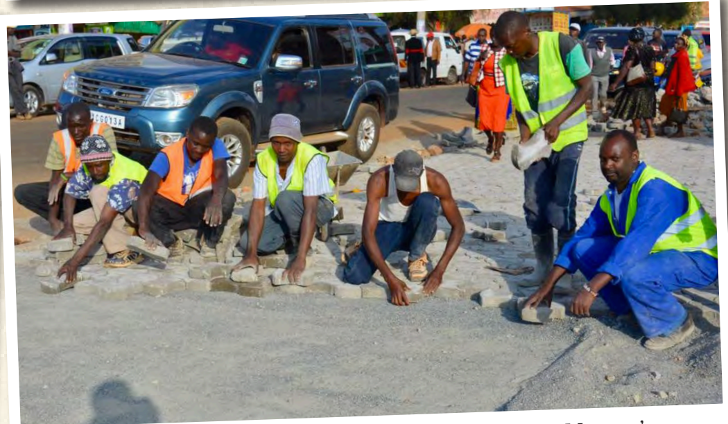
Ongoing laying of paving blocks in Kangema Town, Murang'a
