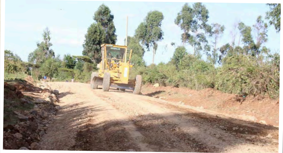
Road construction in Uasin Gishu County
