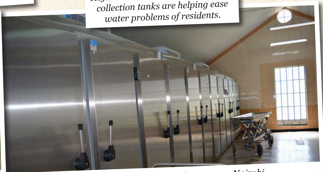
The new Mbagathi hospital mortuary, Nairobi
