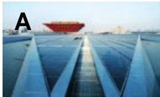
A Shanghai Expo Project-5MW, China
