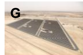
G Masdar solar plant- 5 MW-Masdar, UAE
