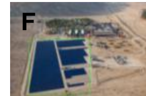
F Ktura solar plant-4.9 MW- Israel
