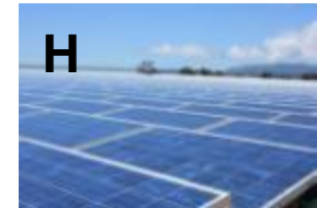
H De Aar solar plant- 100 MW-South Africa
