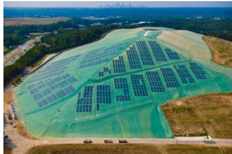
Solar system installed over landfill
