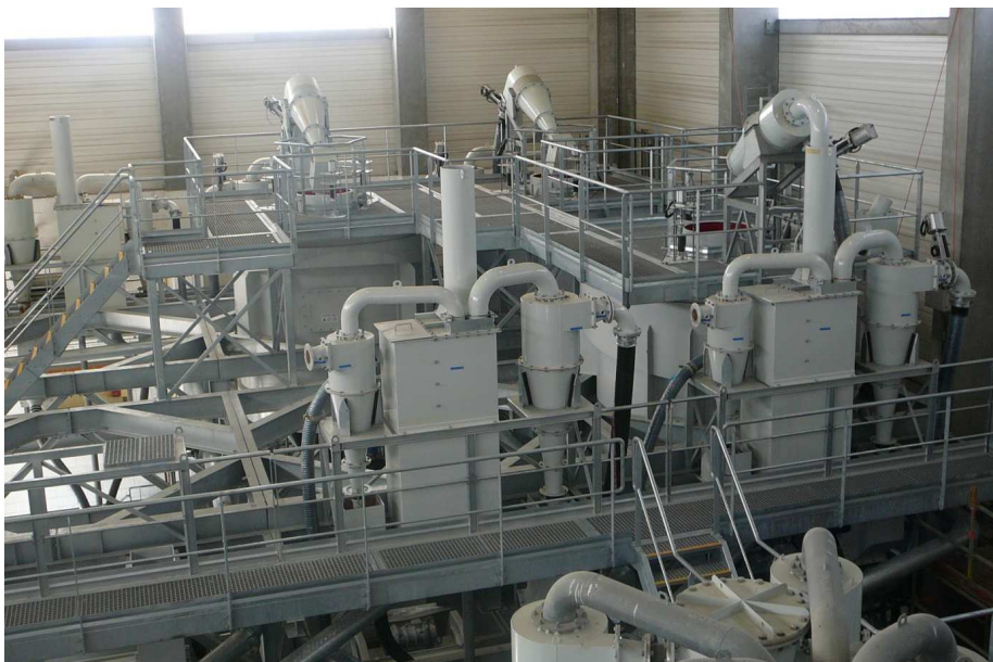
Harbour dredging treatment plant
