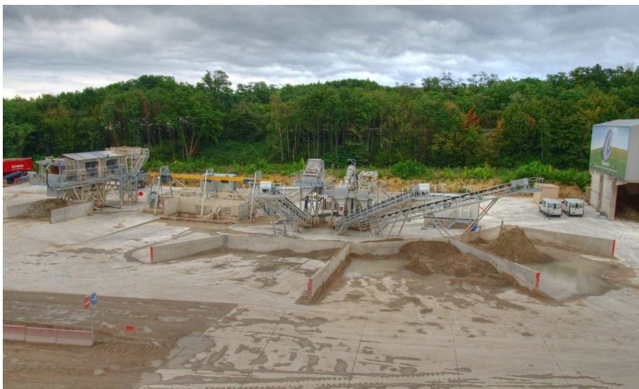
Washing plant for mud residues
