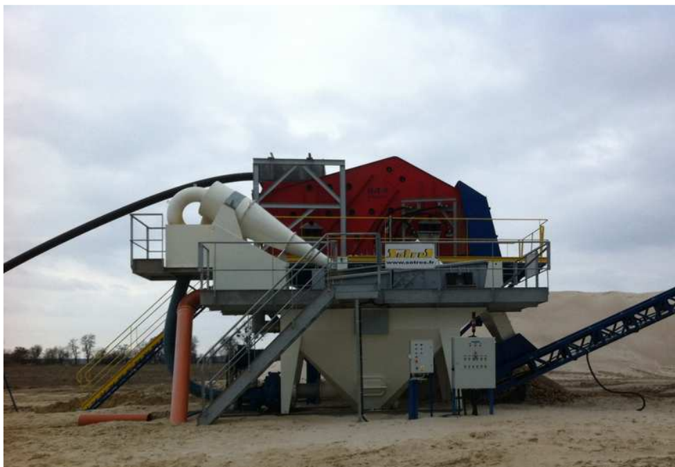
Screen feeded by dredge & sand unit
