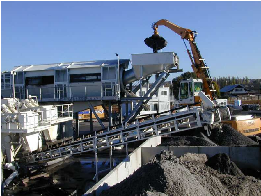
Treatment plant for urban & industrial effluents
