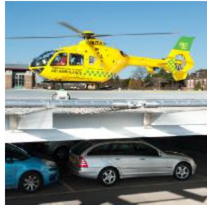
helipad southampton general hospital st.mary's, isle of wight
