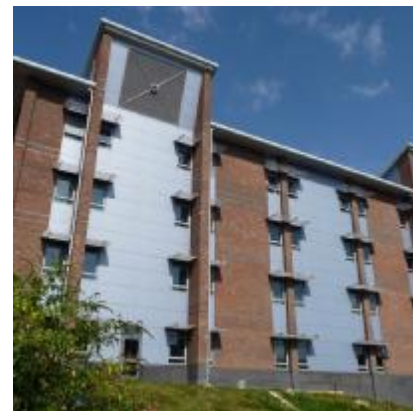
diagnostic treatment centre royal hampshire county hospital
