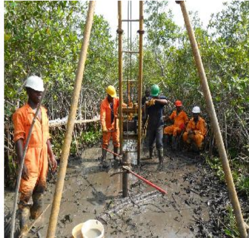
Soil investigation to 15m depth on Road alignment at Ch. 374 + 500
