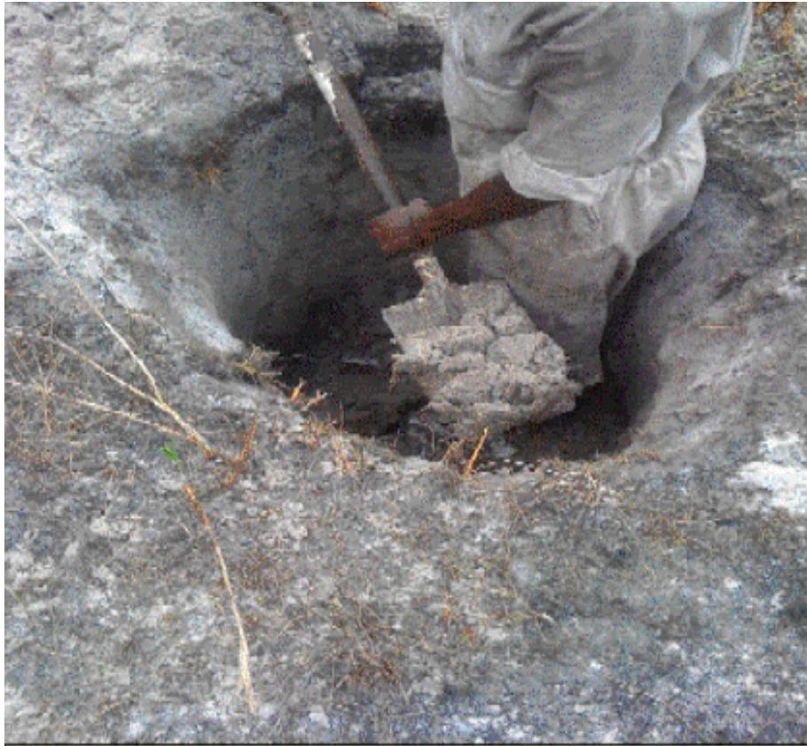
Digging of Trial Pit
