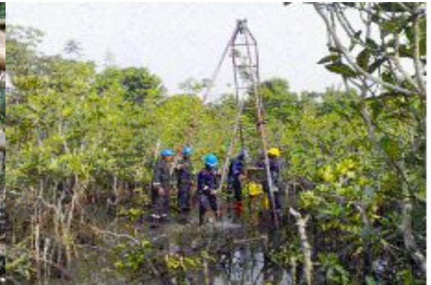
Drilling on the Alignment in Andoni
