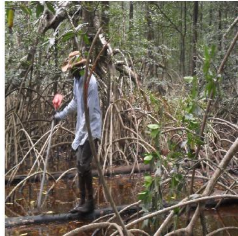
Alignment survey in mangrove swamp in progress about Ch.537 + 100
