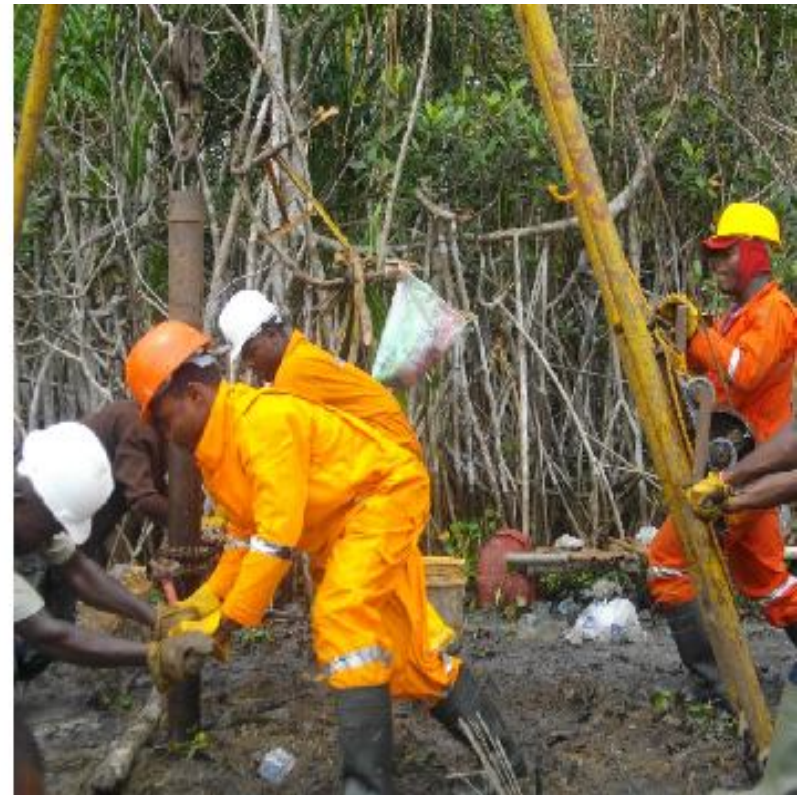
Soil investigation to 15m depth on Road alignment at Ch. 41 + 200
