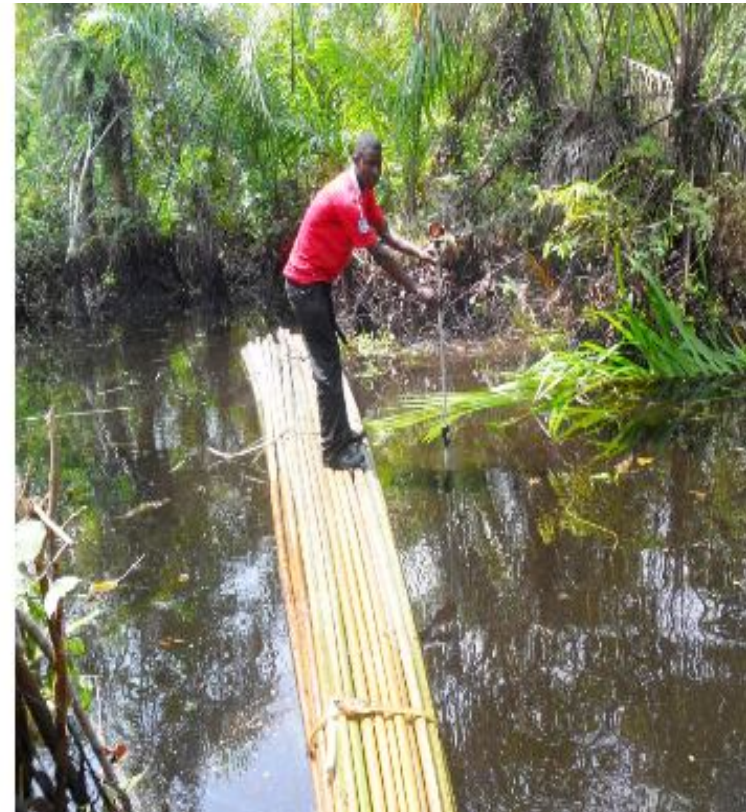
Alignment survey in fresh water swamp in progress about Ch.585 + 300
