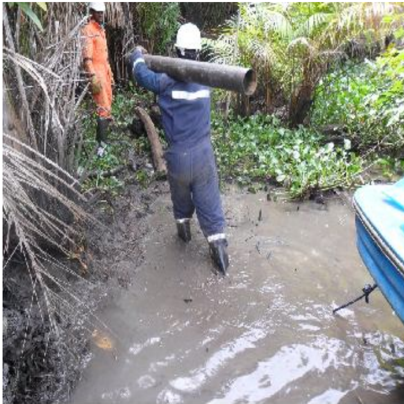
Soil investigation team moving equipment to a test location about Ch.389 + 862.5
