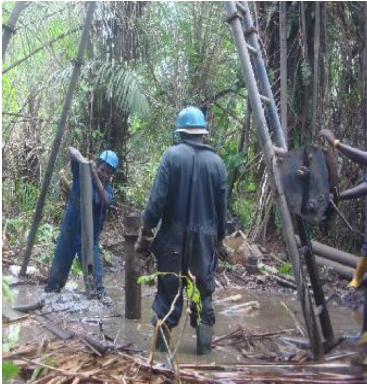
Soil investigation to 15m depth on Road alignment at Ch. 574 + 300
