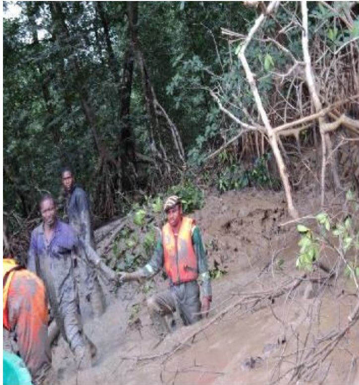
Soil investigation team moving equipment to a test location about Ch. 272 + 325
