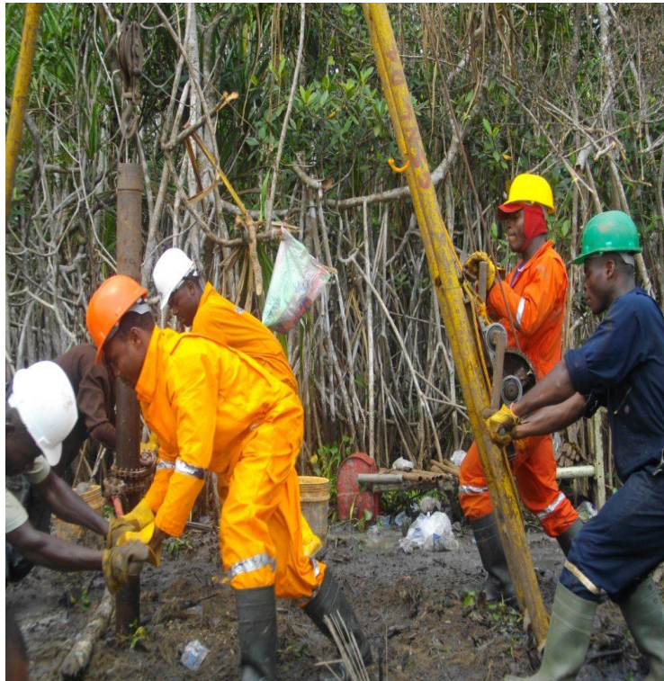
Soil investigation to 15m depth on Road alignment at Ch. 41 + 200
