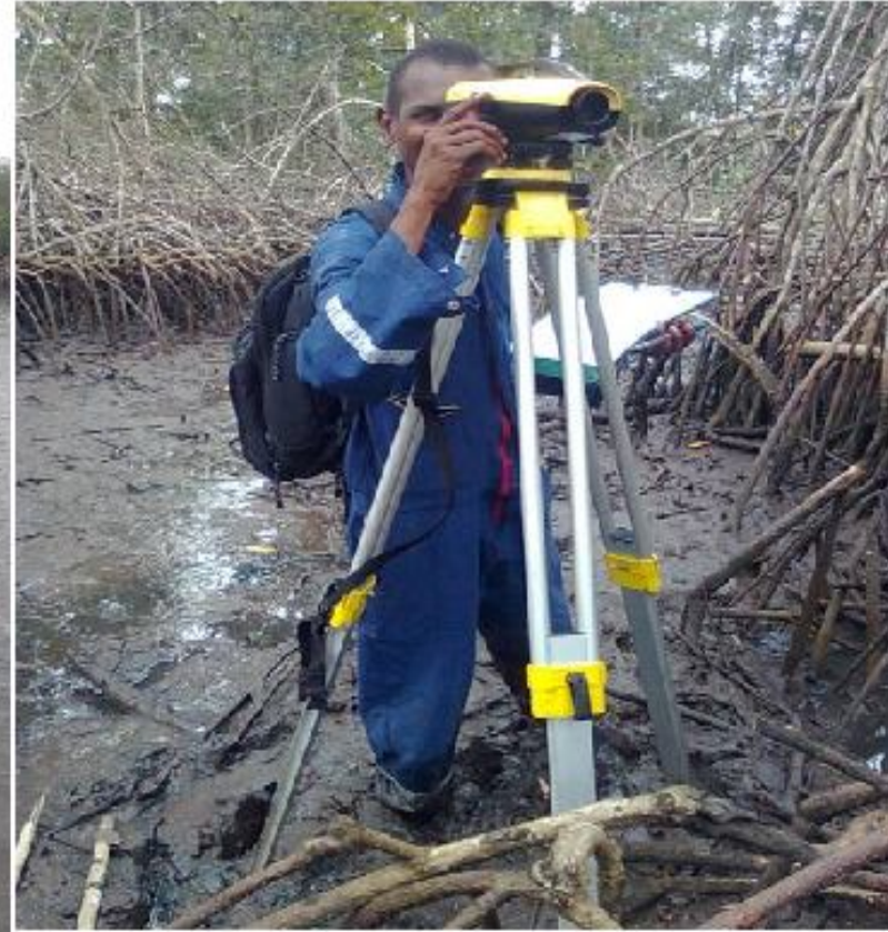
Alignment survey in mangrove swamp in progress about Ch.244 + 900
