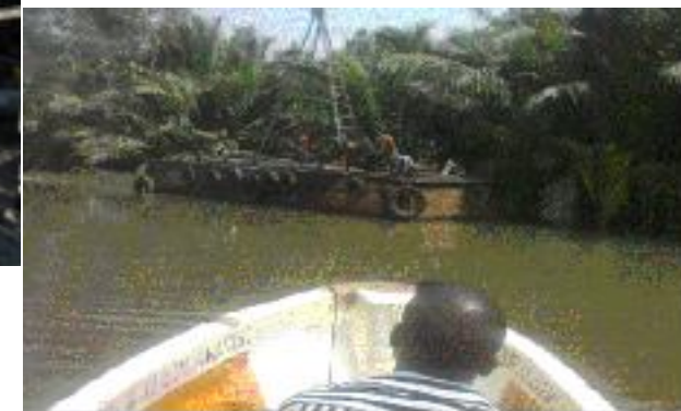
A Barge Mounted Drilling Rig
