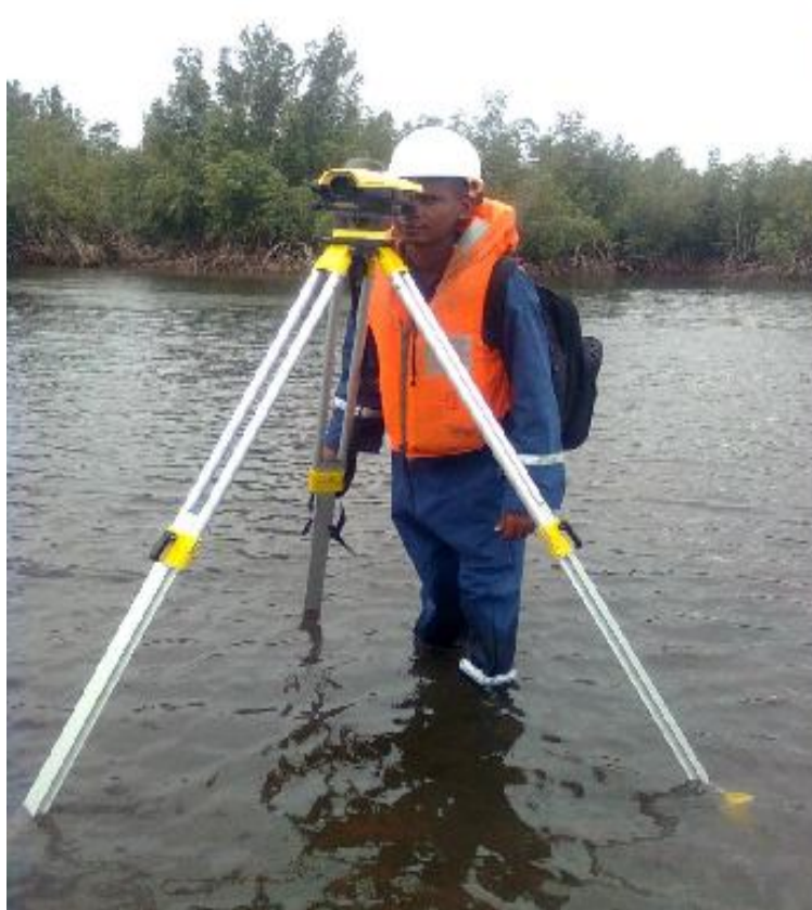
Alignment survey in mangrove swamp in progress about Ch.180 + 700
