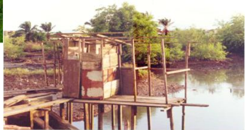
Poor social infrastructure - Pier latrine, common in the study area
