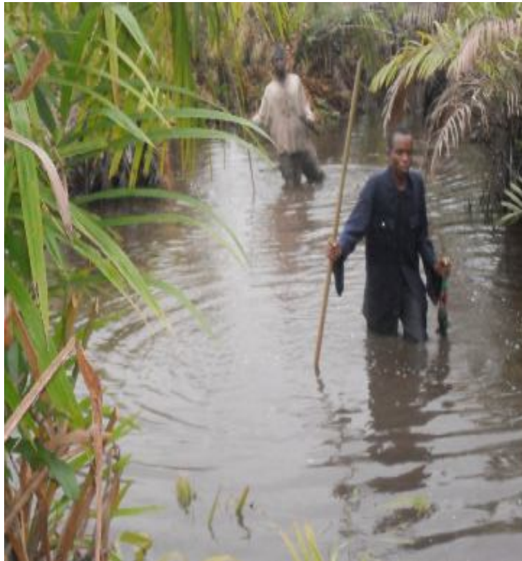
Alignment survey in salt water swamp in progress about Ch. 540 + 300
