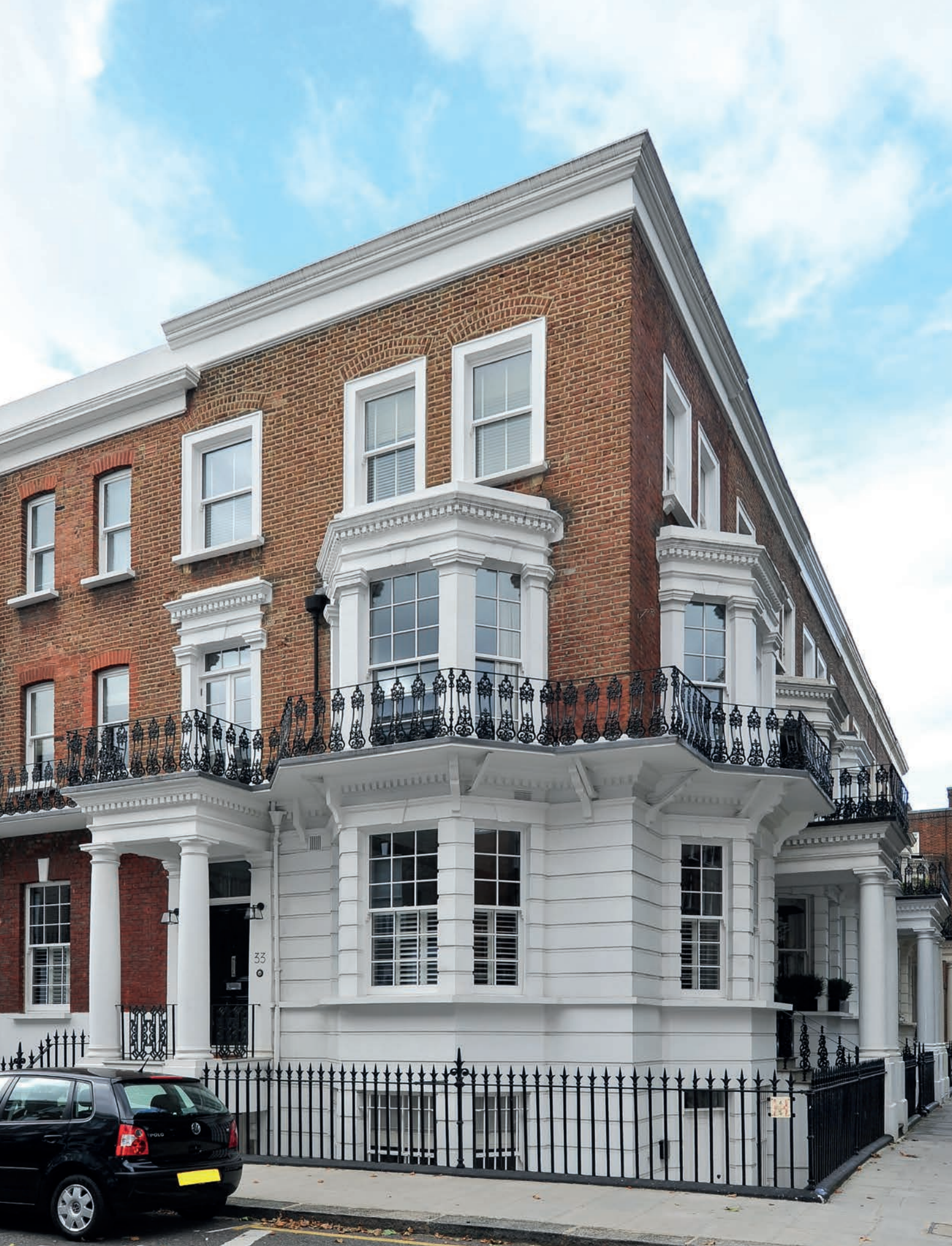
Complete new sash windows manufactured and installed.
