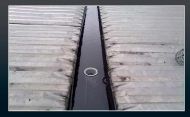
CSC recommend gutter lining is installed to all gutters regardless of age and condition.
