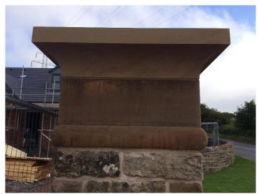
An untreated Buff Sandstone pillar cap that has darkened due to high levels of Manganese within the stone
