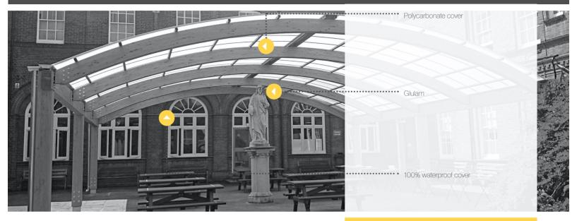
Fordingbridge utilise the industrial wooden product of glued laminated timber (glulam). Glulam is a safe material for nearly all structural tasks that allows for highly variable designs.
