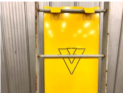
Step 1. Hang guard on ladder
