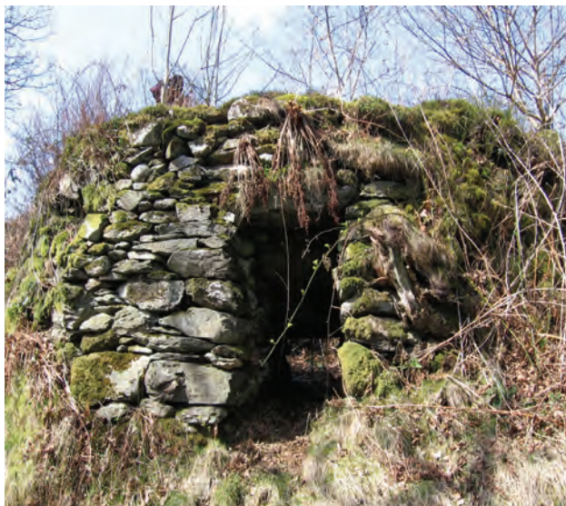
Photo 51 A constructed potash kiln at Stephenson Ground
