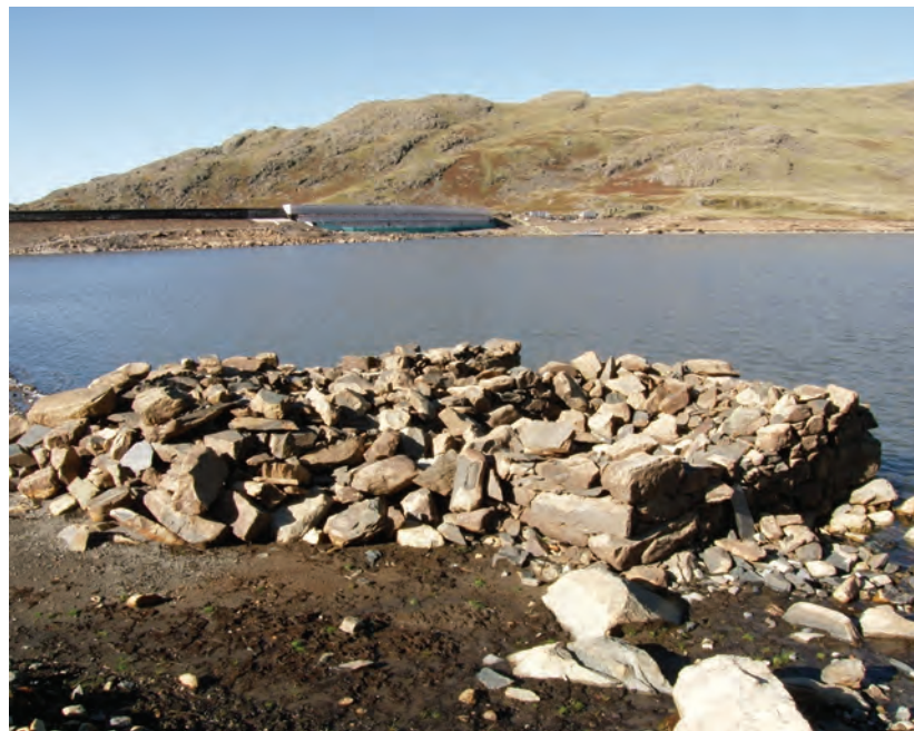
Photo 48 The normally submerged boathouse ruin revealed during the draining of Seathwaite Tarn reservoir. The dam, in the process of repair, is visible in the background.
