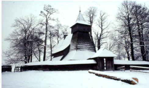
16 th Century Timber Church: Debno, Poland
