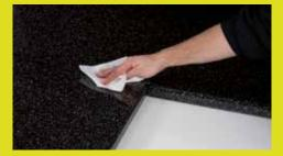
Moisten a clean, lint-free cloth with white spirit and carefully remove the residue, wiping at 90° across the joint to avoid removing adhesive before the joint cures.
