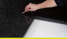
Apply a continuous 5mm diameter bead around the border of one cut edge, 5mm in from the bottom and top faces following the profile and completing a loop. Do not reduce the amount of adhesive recommended.
