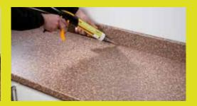
Clean away any spillage with a clean wipe moistened with white spirit. Do not use water or other solvents.
