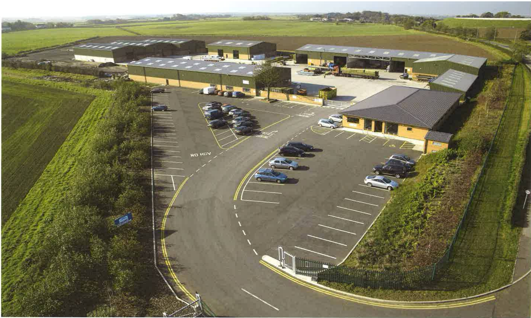
The spacious modern site at Westby is situated on the main A583 within a geographical mile of the original Smithy Fold site at Wrea Green, yet a "million miles" away from the premises that George and James worked in.
