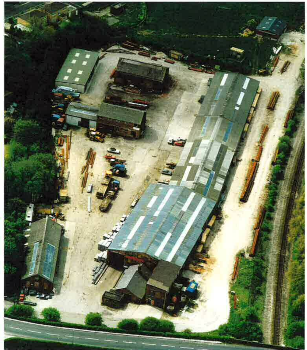
Now showing Brook Mill in mid 1990s with adjoining railway yard being used for steel storage
