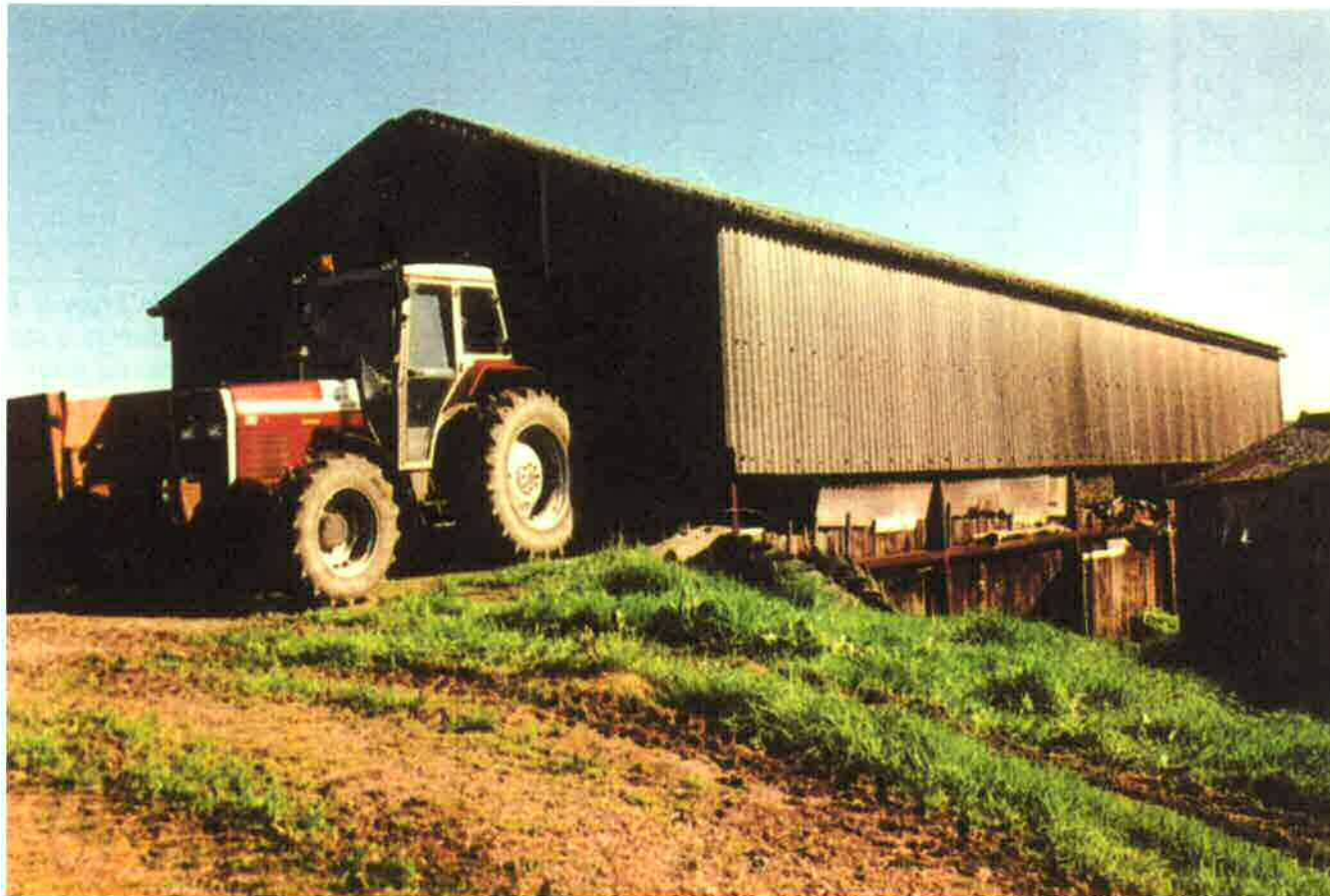
Mr Dixon's building in Cumbria
