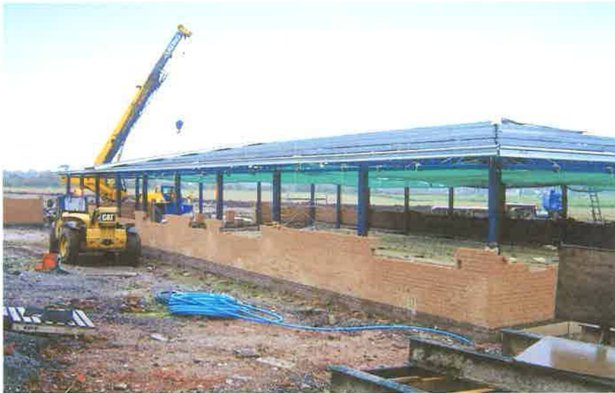
The office block under construction
