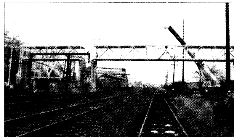
GCRTA Photo Rapid transit is a big lift. Greater Cleveland Regional Transit Authority's new stations create good-paying construction jobs, such as in 2009 when the Puritas Red Line station was under construction next to and over the Norfolk Southern/Amtrak line. After it opened May 17, 2011, the Kamms Corners Development Corp. began creating a Transit-Oriented Development guideplan for this station and the next station east at West Park.
