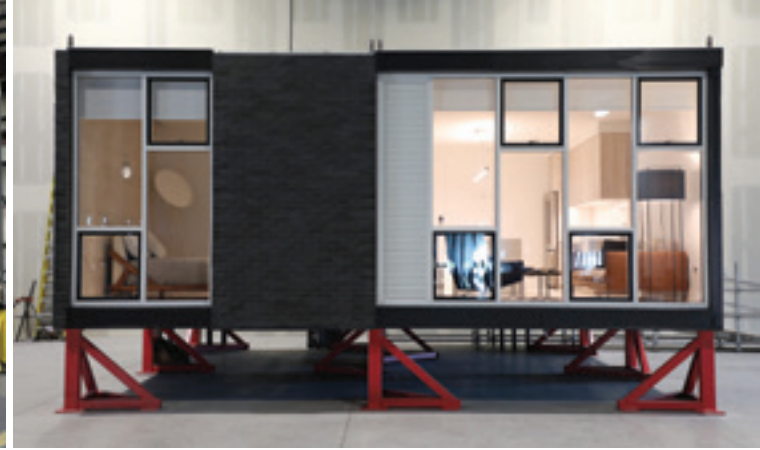
Modular units can be constructed indoors, limiting weather-related delays and improving quality control.
