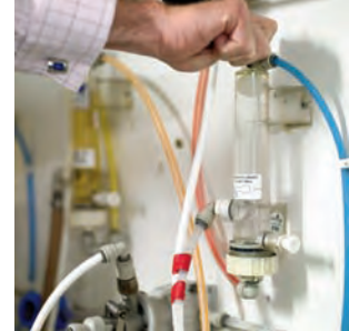
3. Switch on gas supply to cleaning bottle and flush beer from cellar buoy with fresh water
