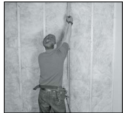
Measure the height of the wall
