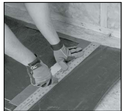
Cut Barrier to the appropriate length.
