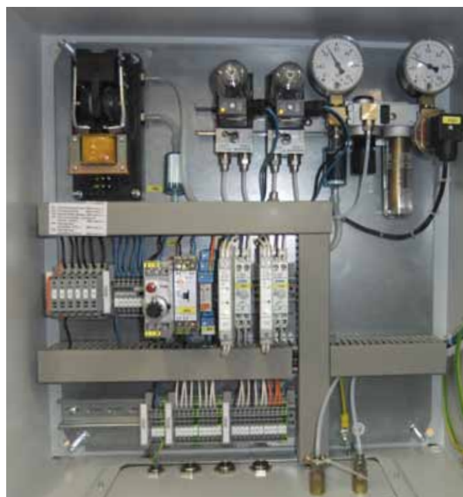
Reference Air Unit with pressure control valve and Air Pulsing Unit
