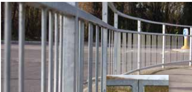
Staggered infill bars (above),
