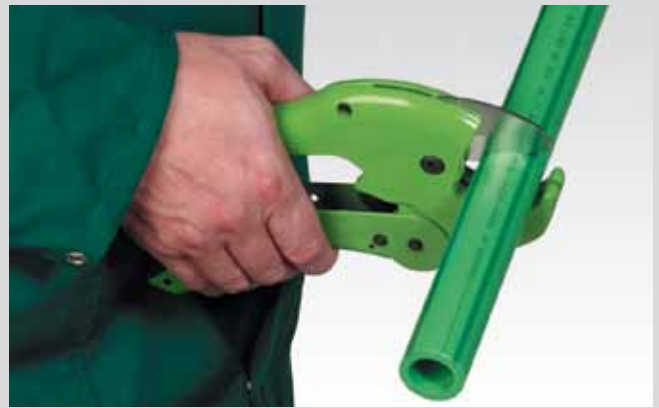
Cutting of the pipe
