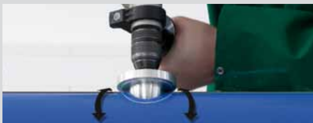
Removal of the oxygen barrier layer from the aquatherm blue OT-pipe
