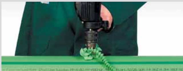
Drilling through the pipe wall
