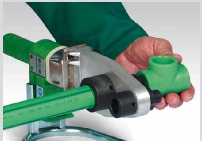
Heating-up of pipe and fitting
