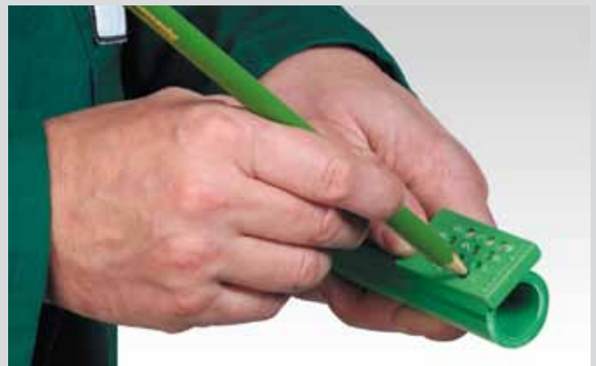
Marking of the welding depth
