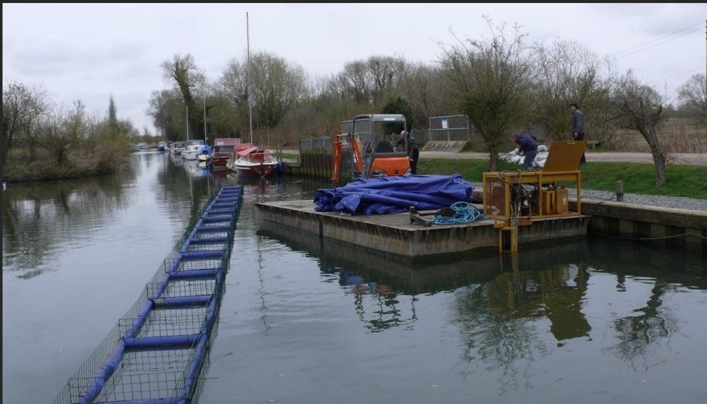
Systems unloaded at Rockland Staithe ready for the short trip up to the Broad
