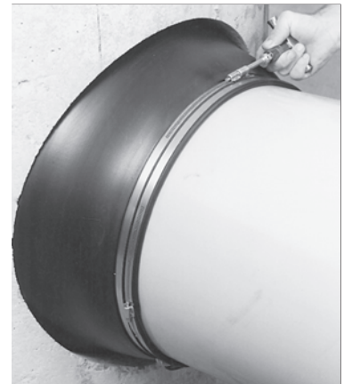
Install Pipe Clamp(s) with T-Handle Torque Wrench
