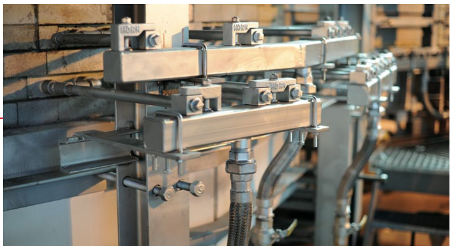
Double burner manifold Gas / air mixture burners
