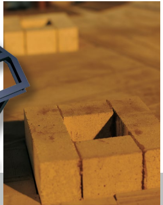
Waste gas openings
