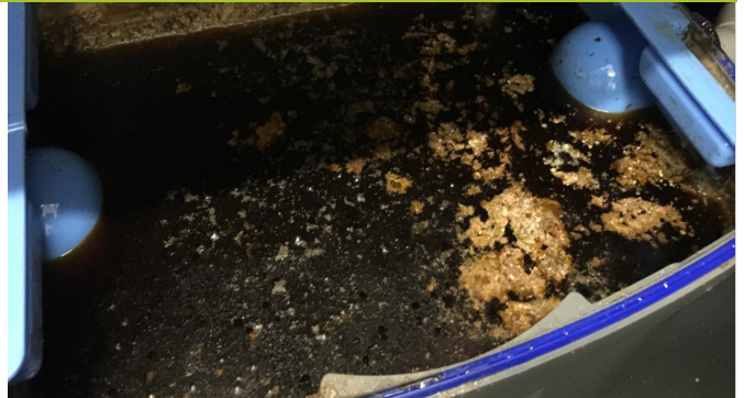
21 September 2017 - 27 days with bio-dosing. More sediment in bottom of F.I.T unit, but barely noticeable.
