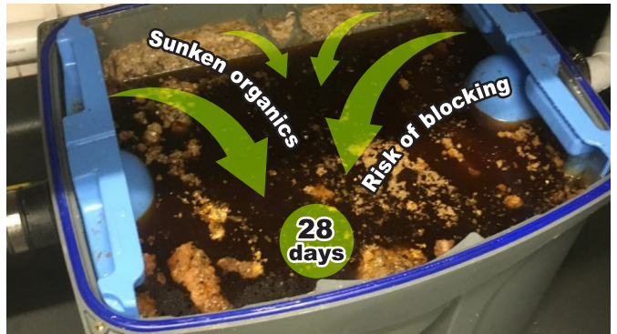
25 August 2017 - 28 days in. Floating organics had become saturated and sunk, leaving around 10mm of floating oil. The unit was completely full – 40 litres of organic material and 10 litres of oily water were removed.
