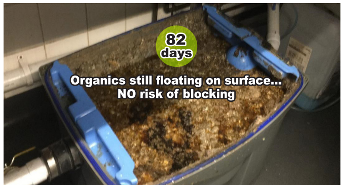
15 November 2017 - 2 days short of 12 weeks. 5 litres of floating organic material, 5 litres of sunken food/organic waste debris and 40 litres of oil and water were removed. End of trial.
