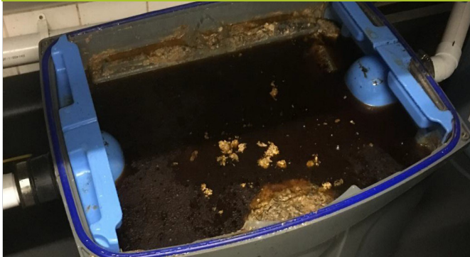
5 September 2017 - 11 days with bio-dosing. No floating organics. Small amount of sediment in bottom of F.I.T unit (by-product of FOG degradation).
