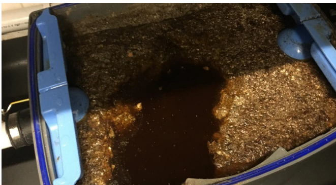
6 October 2017 - 32 days with bio-dosing. Floating organics, but only a few mm thick.
