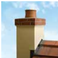
Brick or Stone Chimney (Class 1) 1
