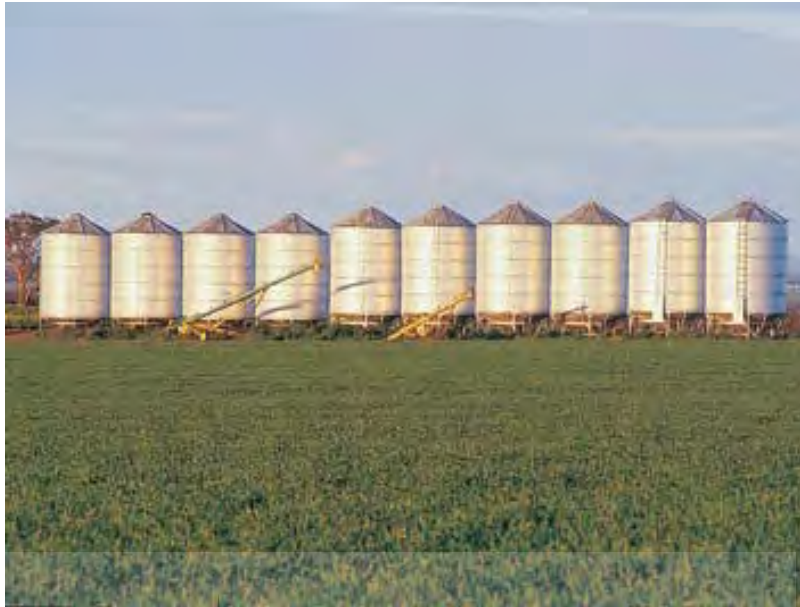
Figure 12: A photograph of bolted steel silos which are commonly used for grain storage (Viljoen, 2001).
