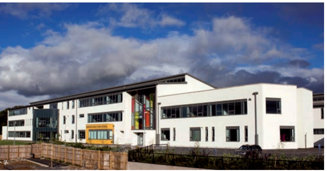
Education (1) Ashfield Girls' High School, Belfast, main approach (2) Ashfield Girls' High School, Belfast, entrance hall (3) Ashfield Girls' High School, Belfast, rear elevation detail (4) Ashfield Girls' High School, Belfast, atrium detail
