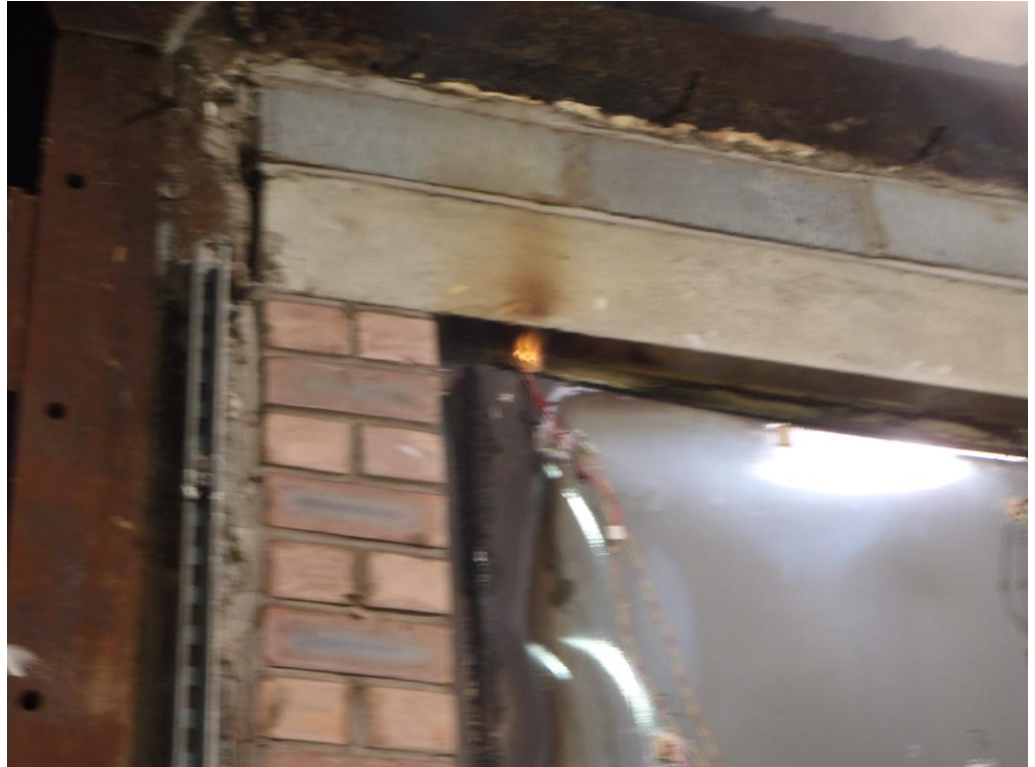
Sustained flaming integrity failure of Doorset A after 34 minutes of testing
