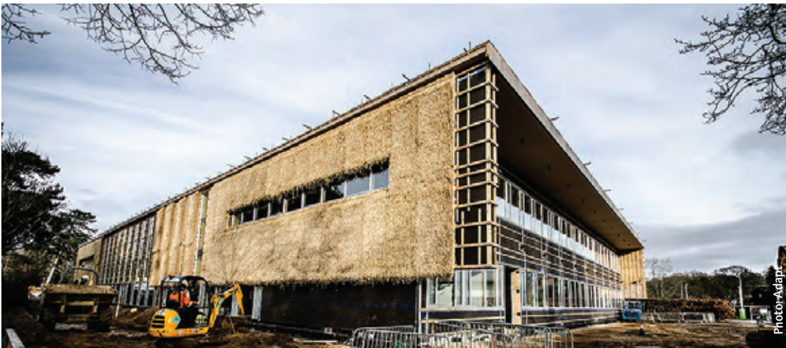
Thatch cassette installation. Photo: Adapt
