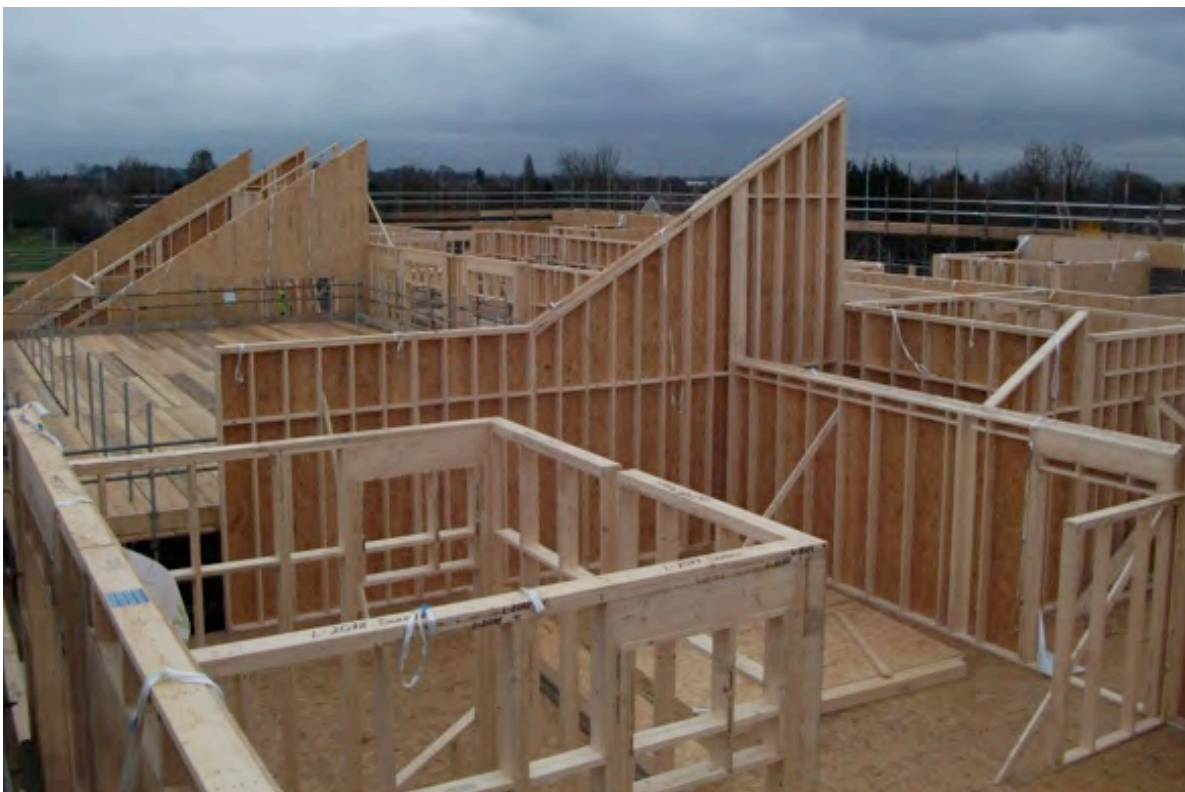
Lightweight timber frame construction – Oakmeadow Primary School Photo: Architype
