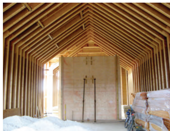
BELOW: I beam portal frame Photo: Conker Conservation
