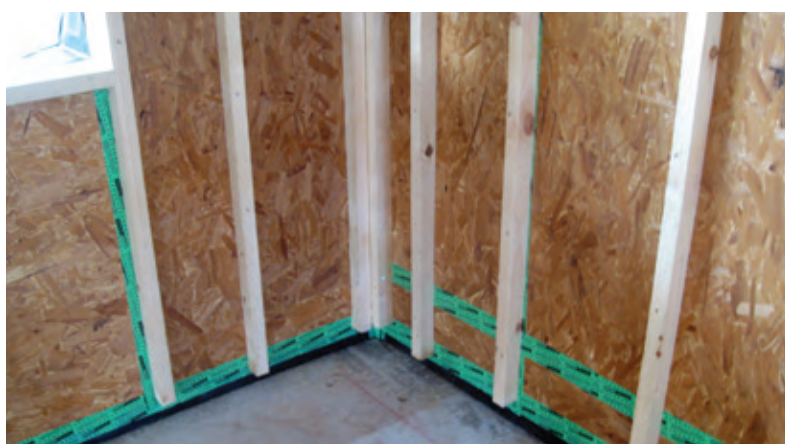
ABOVE: 18mm OSB-3 with joints taped successfully installed as airtight membrane. Photo: Eco Arc Architects
