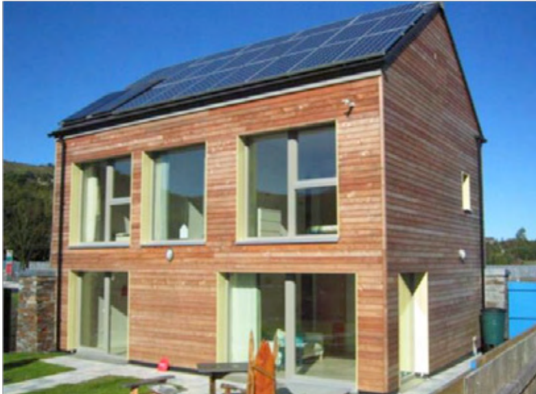
Larch House, Ebbw Vale, using both PV and Solar thermal Photo: bere:architects
