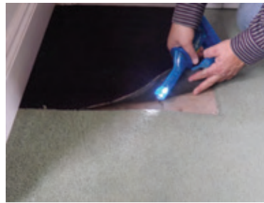
Using chemical smoke to check for leakage between upper floorboards
