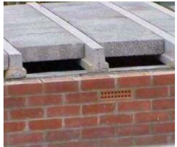
ABOVE: Beam and block floor construction Photo: Green Building Store
