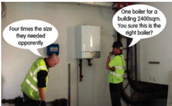
BELOW: Passivhaus reduces the need for services! Photo: Nick Grant
