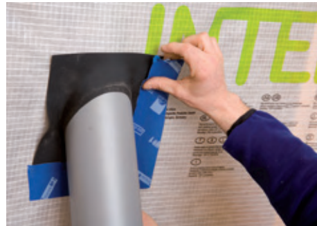
LEFT AND RIGHT: Sealing pipes and cables. Photos: Ecological Building Systems
