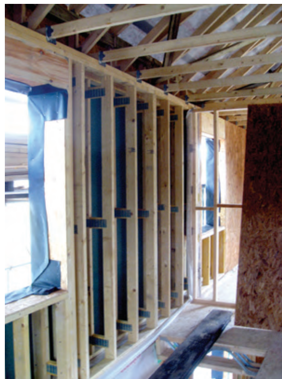
ABOVE: Larsen timber trusses Photo: Eco Arc Architects
