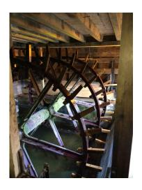
This is the waterwheel with all the old timber removed. The replacement I" thick oak boards, were purposefully left raw to prevent any treatment from leaching out into the river and harming the wildlife.
