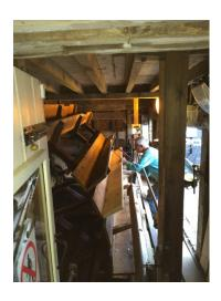
Each of the 30 floats were carefully added, working evenly around the wheel to maintain balance. Because the ceiling beam has dropped over the decades, a piece of each float had to be removed to provide clearance.
