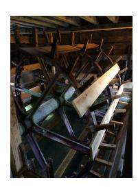
The rebuilding of the waterwheel began with the 90 oak Starts being fitted. The Backboards were then fitted between the Starts, ready for the floats (also known as paddles) to be attached.
