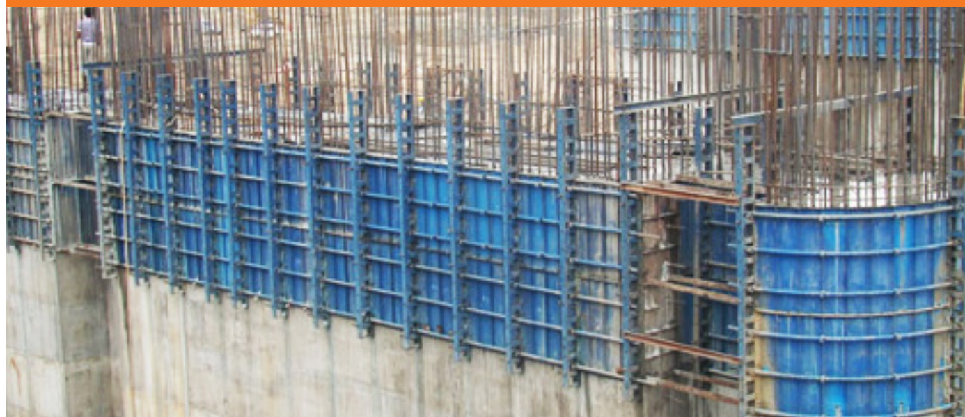
SHUTTERING FOR BARRAGE
