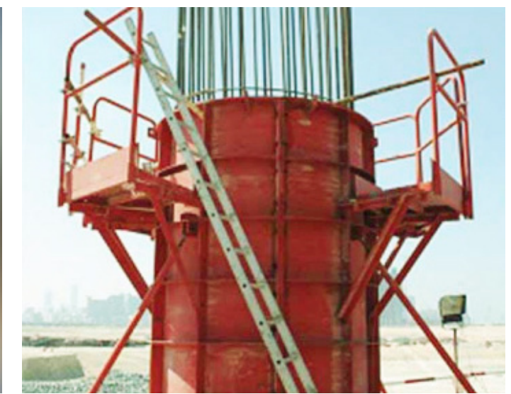
Pier Formwork
