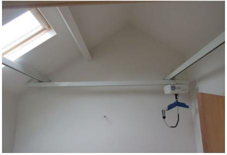
Large H system fitted on wall brackets
