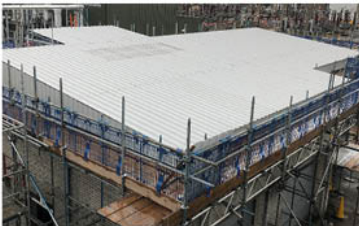
top left : View of FTP completed with single skin steel sheet
