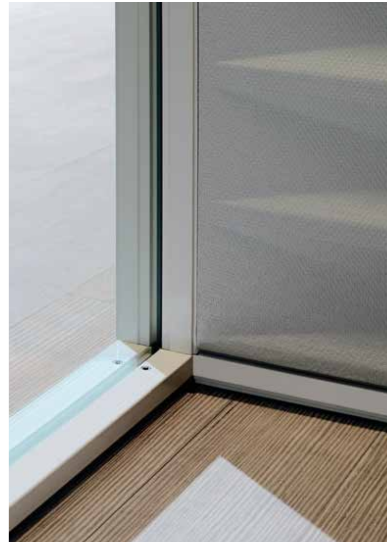
Internal corner junction
