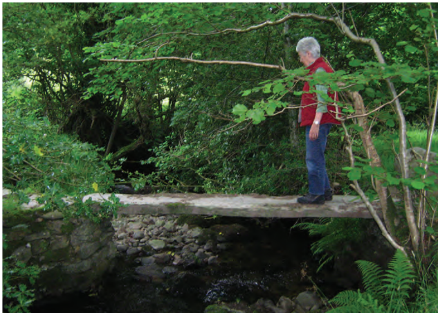
Photo 16 ( Above ) Birks Bridge – built as a pack horse bridge
