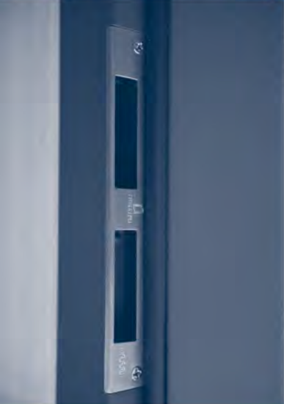
Radiused Strike plate recessed and fitted onto frame
