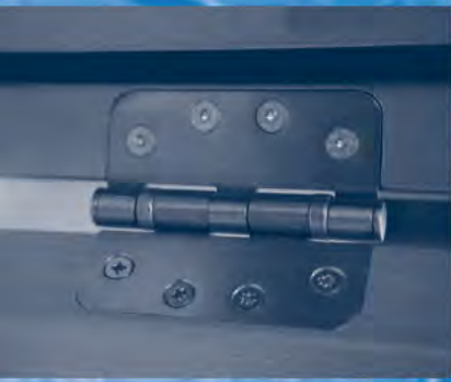
Recessed radiused type hinge fitted onto Steel frame and timber door.
