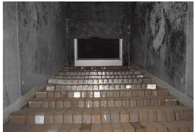
Figure 4.33 Moving grate in an overfed stoker boiler
