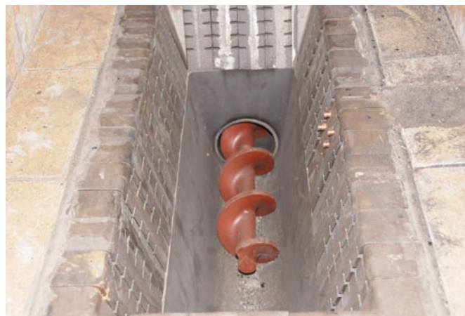
Figure 4.8 Underfed stoker grate
