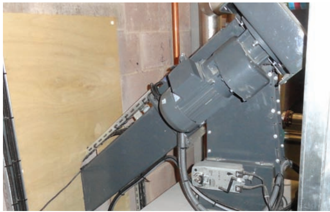
Figure 3.15 Rising auger showing rotary valve in fuel feed system
