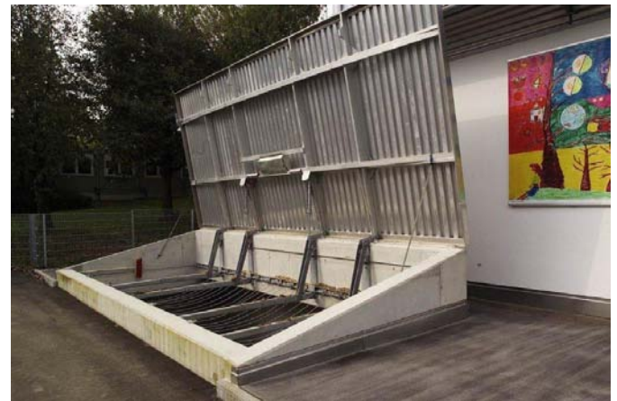
Figure 3.4 Underground silo showing lid and safety grille
