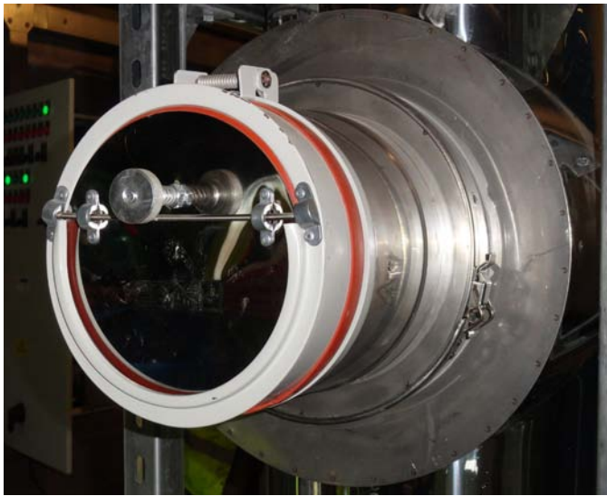
Figure 10.2 Combined draught stabiliser and explosion relief panel
