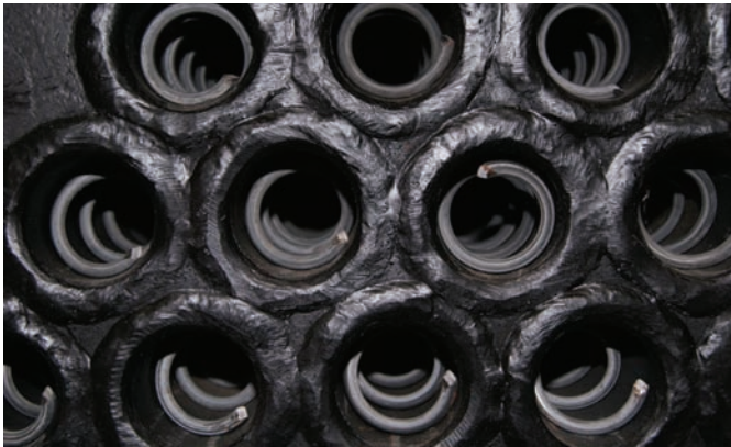
Figure 4.18 Horizontal fire tubes
