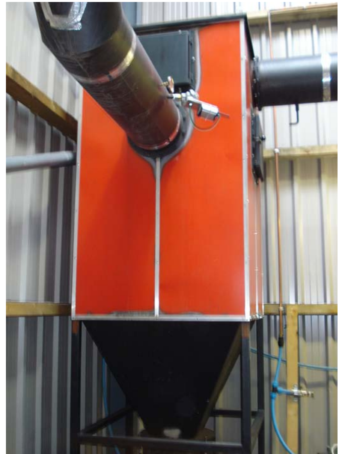
Figure 4.40 Cyclone grit arrestor
