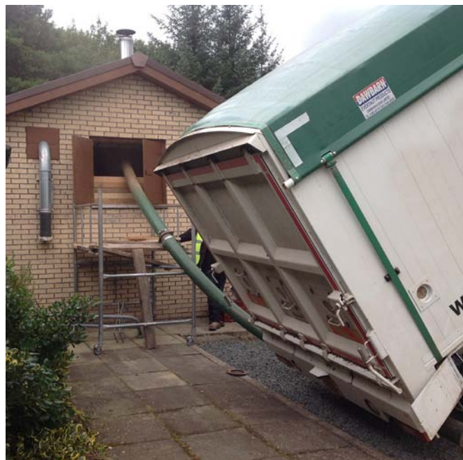
Figure 3.2 Blown delivery of woodchips
