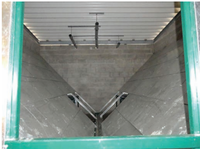
Figure 3.14 V-shaped pellet floor under construction showing fuel fill pipes at top
