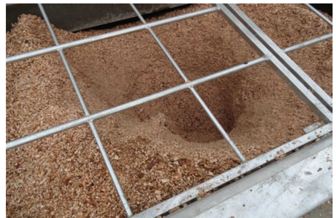
Figure 3.5 Close-up showing the safety grille on an underground silo
